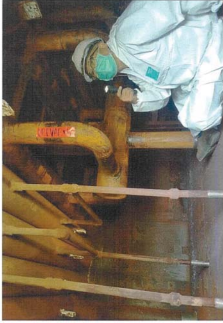
Inspect LP Evaporator Header
