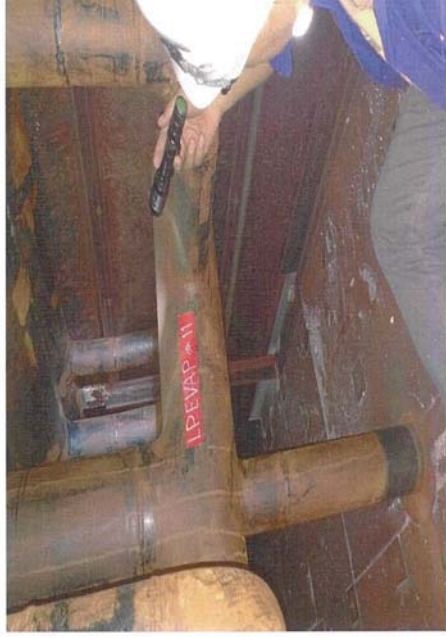
Inspect LP Evaporator Header
