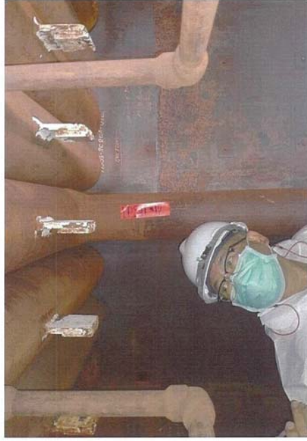
Inspect LP Superheater Header
