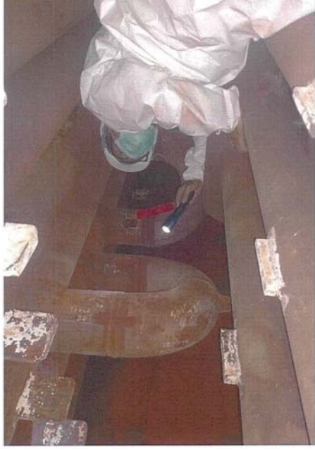
Inspect HP Superheater Header
