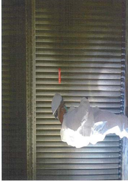
Inspect LP Economizer Tube Panel
