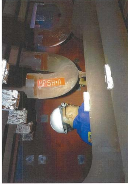
Inspect HP Superheater Tube Panel
