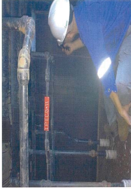
Inspect LP Economizer Tube Panel
